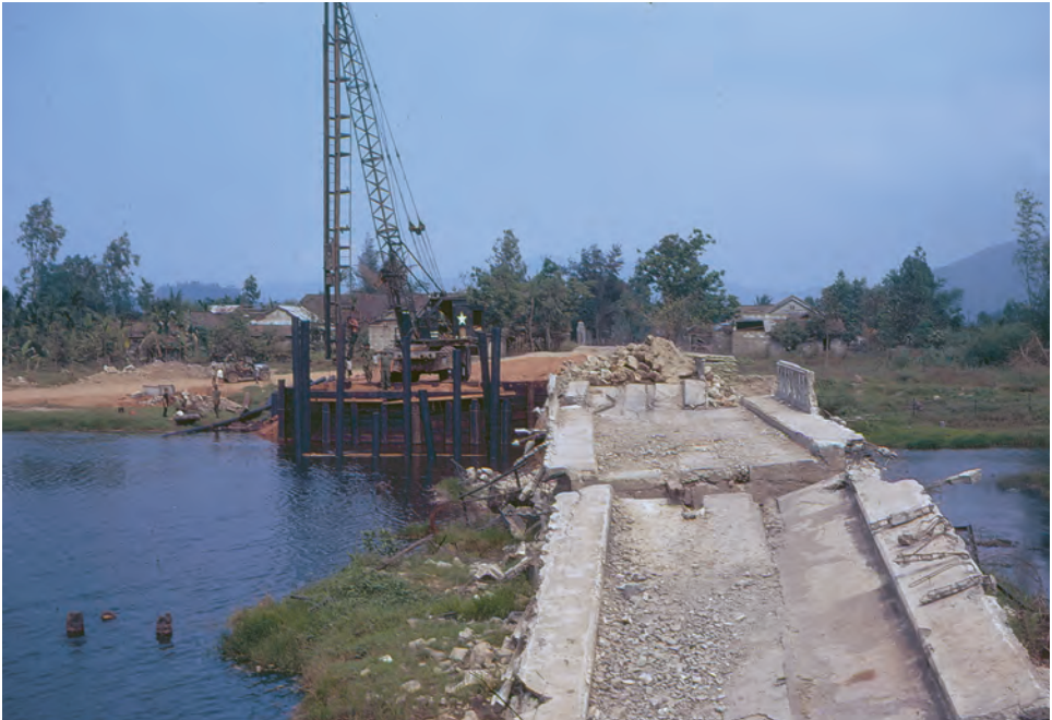
North of the Hai Van Pass, the enemy destroyed bridges like this French-type concrete bridge.
